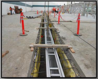
Bodies can be fabricated in the shop in lengths up to 40' and can be fitted together with either flanges and neoprene gaskets or field welded. End and bottom outlets are included.
